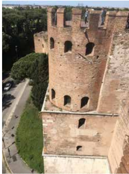
Fig. 3. Masonry of San Sebastiano Gate.
